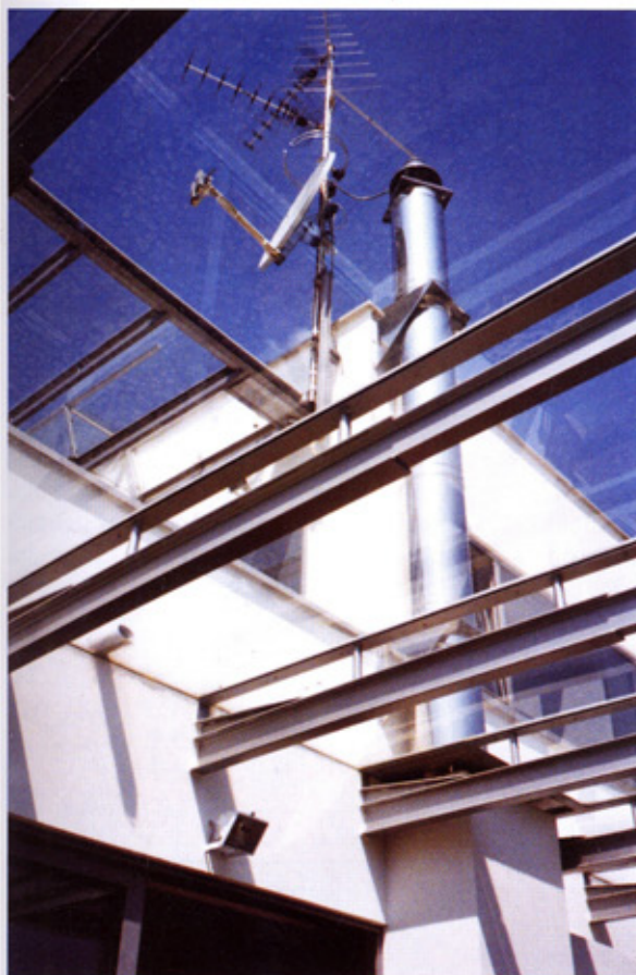
Slika 7: Ostakljene nadstrešnice i dimnjak kamina. The glazed overhanging roof and fireplace chimney.
