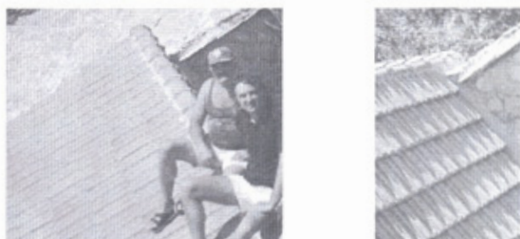
Fig. 8 – Roof is finished: it looked as a well-done job, but...!
