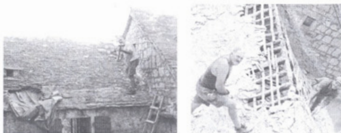
Fig. 6 – Beginning of work-taking stone tiles from the roof down
