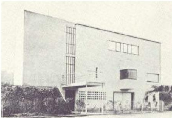
Fig.1.Vaucesson -the Le Corbusier's first modern villa from 1922.
